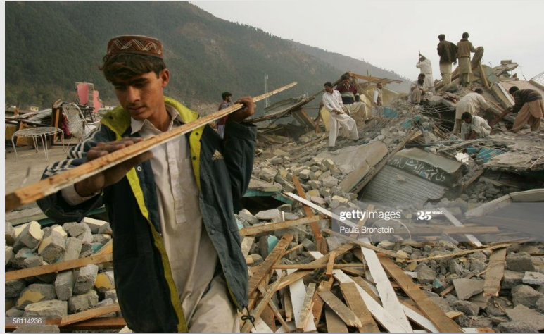
a worker helps to clear the debris.
