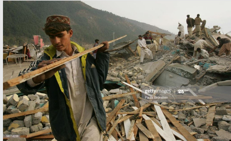
a worker helps to clear the debris.
