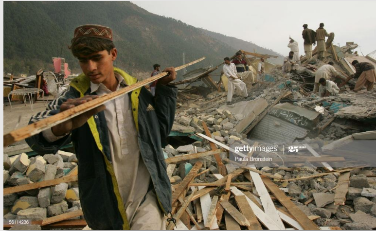
a worker helps to clear the debris.
