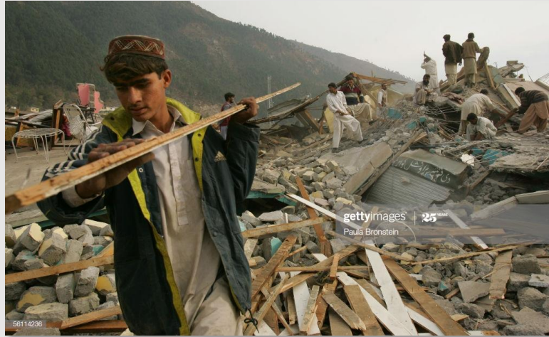
a worker helps to clear the debris.
